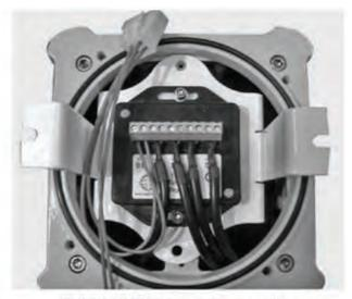
SL10 AMP Regulator shown when correctly fitted
