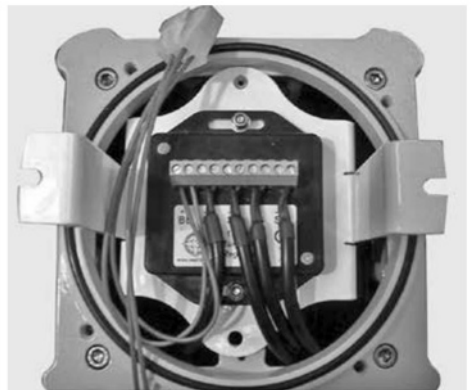
SL10 AMP Regulator shown when correctly fitted
